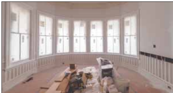
New windows and trim have been installed in a room looking out over Short Beach.
